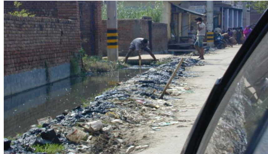
Human exposure to sewage. Muck from the drains being manually removed. Photo:24th Oct. 05, RS.
